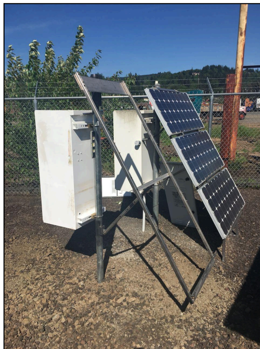
Figure 13: PV Panel stainless steel frame
