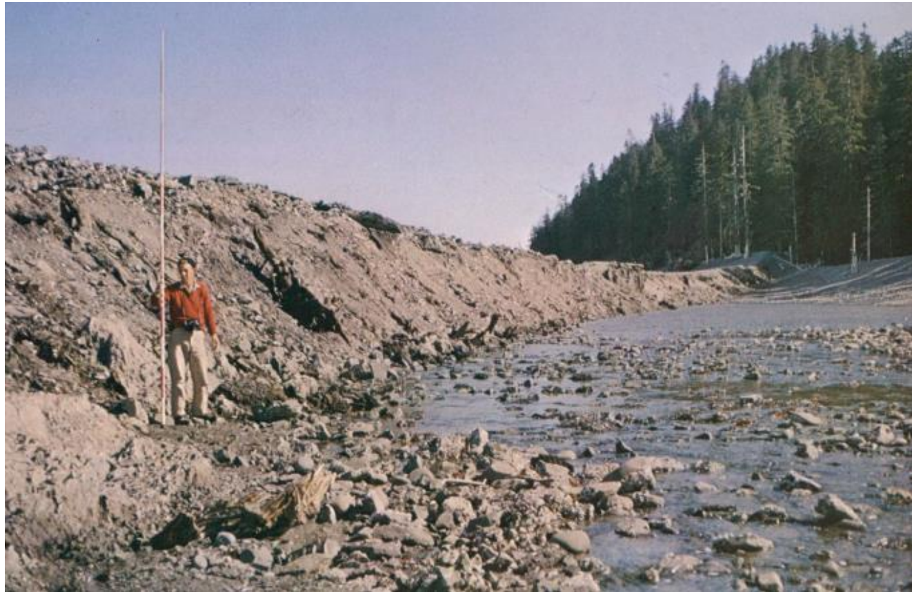
Photo from U.S. Geological Survey Professional Paper 541 The Alaska Earthquake March 27, 1964 Field Investigations and Reconstruction Effort , US Government Printing Office, 1966.
