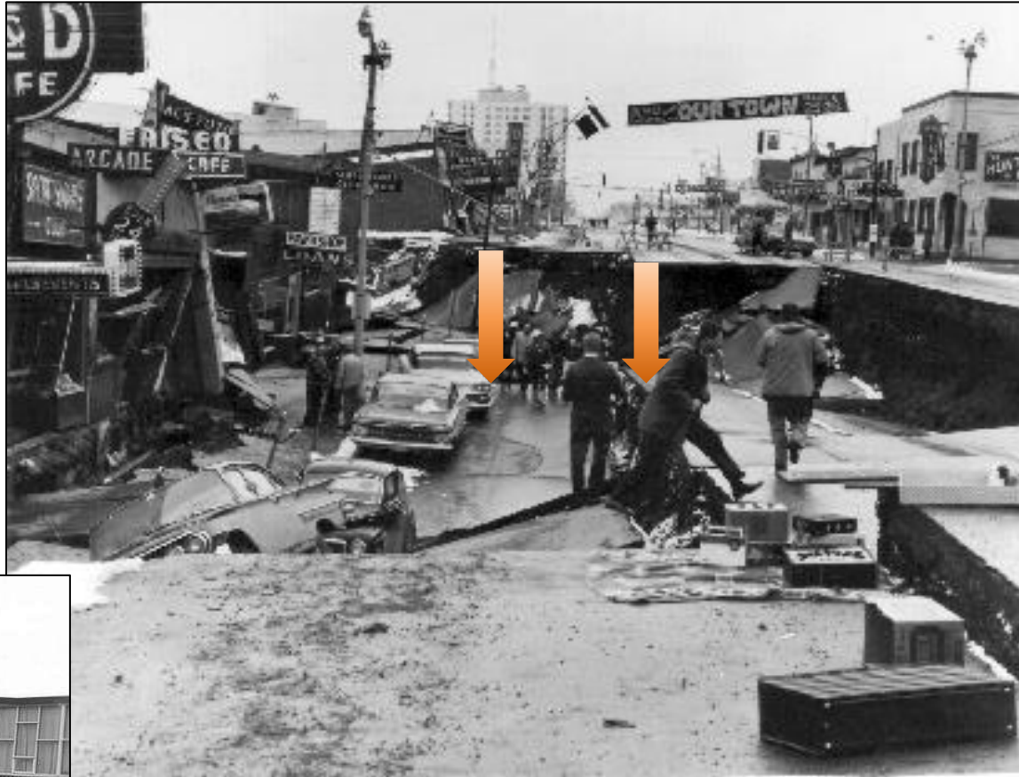
Above: Collapse of Fourth Avenue near C Street, Anchorage. Before the earthquake, the sidewalk and street at left was at the street level on the right. The ground on the left subsided 3.4 m (11 ft) in response to 4.3 m (14 ft) of horizontal movement to the left.
