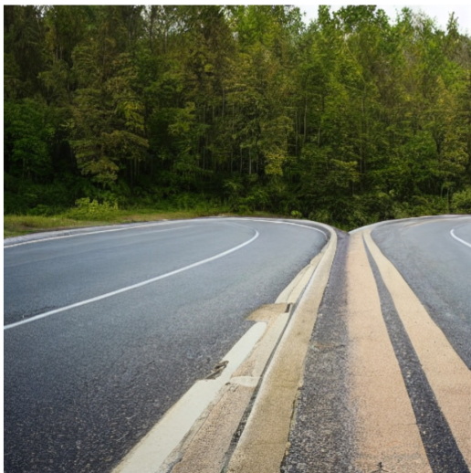
“A road diverging in two different direction”
