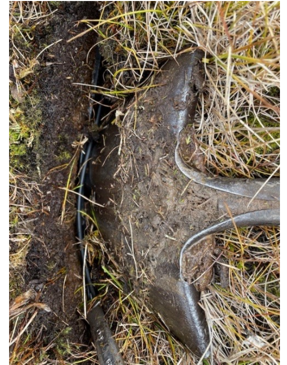
Cable embedment using shovel
